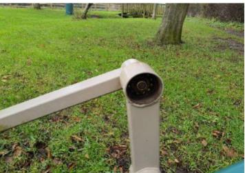
**Finding:** There is / are post or end caps missing / damaged **Action:** Replace missing / damaged post or end caps on the item
