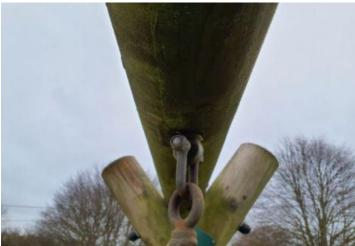
**Finding:** The suspension member shackle is not aligned correctly with the direction of travel creating accelerated wear
