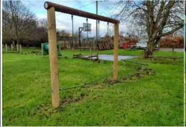
**Finding:** The projecting tree root forms an projecting obstacle / hard object within the falling space of the equipment, in contravention of the requirements of BS EN 1176 Part 1
