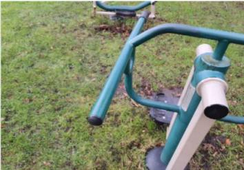
Finding: One or more handgrip(s) are damaged or missing. Action: Replace missing or damaged handgrips
