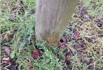
**Action:** Monitor for any deterioration (rot) and replace as required
