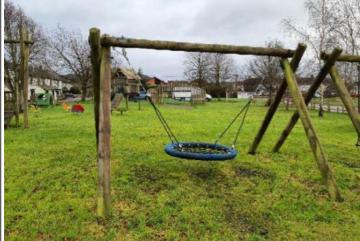
Finding: The ropes/nets are worn/damaged in places
