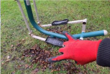
**Finding:** The surface has eroded in some areas and may be **Action:** Reinstate the surface slippery in wet conditions
