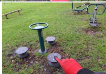
**Finding:** The deflection of the rotating user station exceeds the maximum 105 degrees required by BS EN 16630
