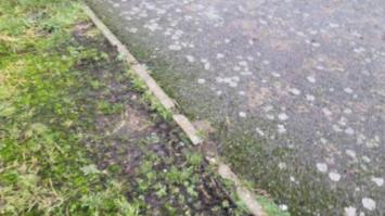
Finding: There are trip hazards at the edges of the surface Action: Remove trip hazard
