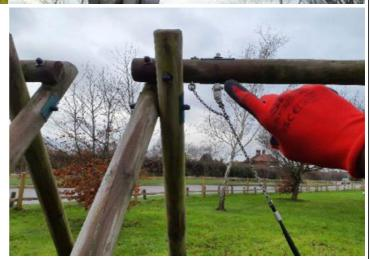
**Finding:** A number of fixing(s) have worked loose on the suspension brackets
