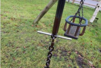
**Finding:** The connecting links are in excess of 8.6mm and less than 12mm and fail the requirements of BS EN 1176 **Action:** Monitor - No action given the risk assessment Part 1; clause 4.2.13, Chains
